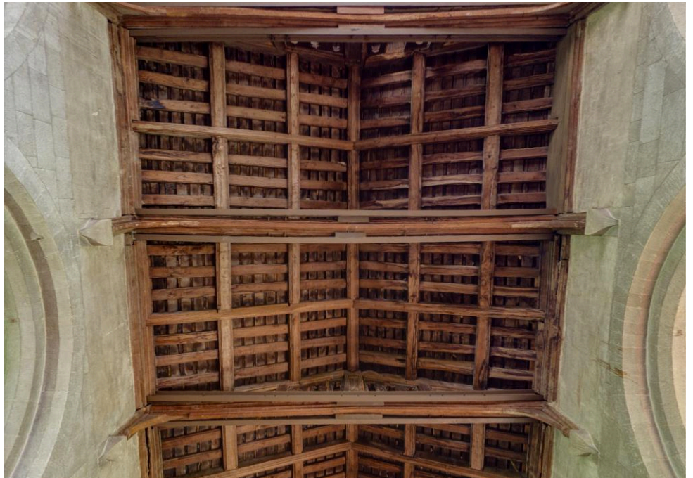
St Andrew's Shrivenham, strengthened roof structure. Photo by Nikhilesh Haval
