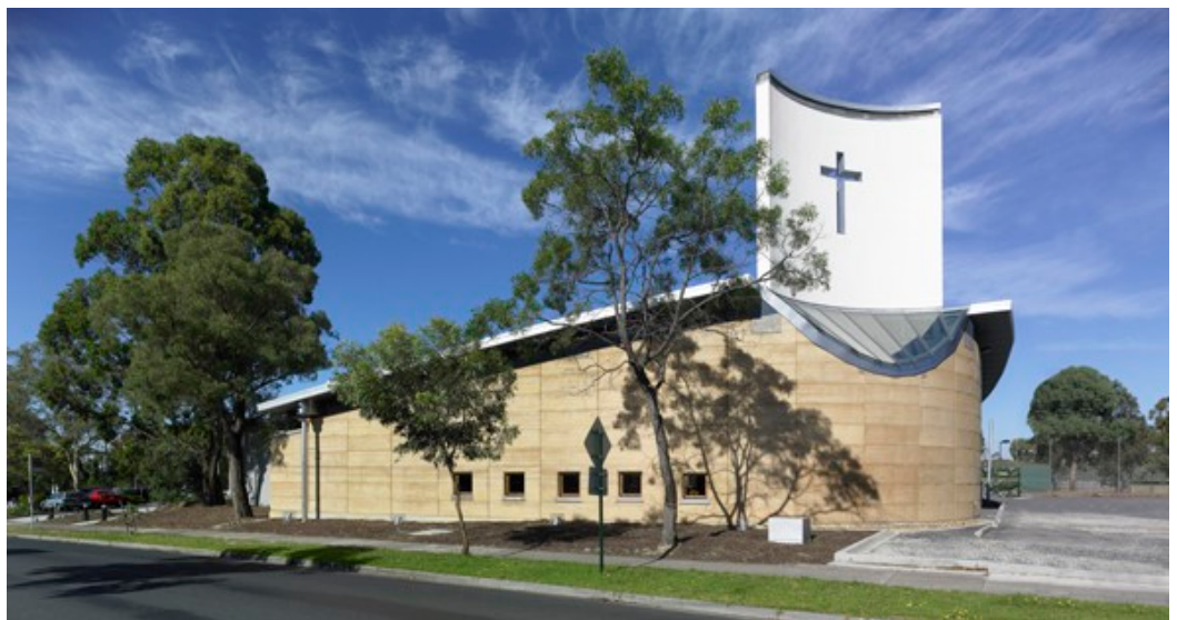
St Alfred's has a solar chimney that uses the sun to draw air out of the auditorium, pulling cool air in from below ground, avoiding the need for air conditioning as well as creating a community focus
