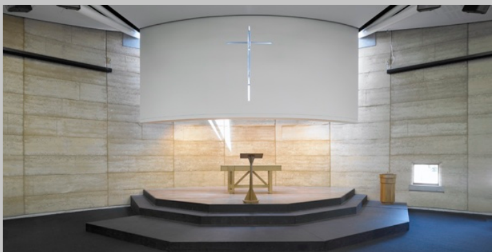
The base of the north blade hangs over the platform. Air is drawn around and below the blade and into the thermal chimney flues on the back. The reflected light source creates a focus for the auditorium.
