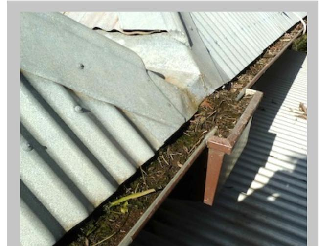
*This gutter & hopper head is on an unused heritage building. Out of sight and out of mind. It needs an overflow "pop" to show when it needs clearing to people below, before the timber backing rots away.*
