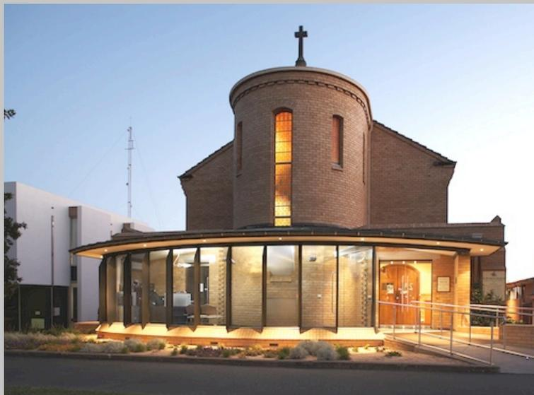
*The thermal mass of the existing brickwork warms-up from the low winter sun penetrating through the new glass at St Peter's Box Hill.*
