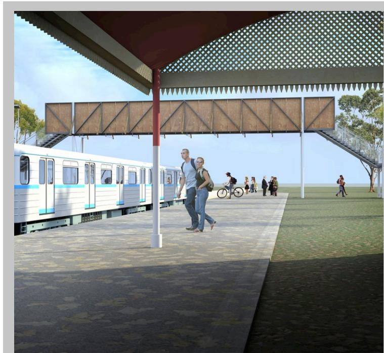
*The replacement footbridge by Studio B at Moorland Railway Station will be a contemporary design based on diagonally braced girder principles.*
