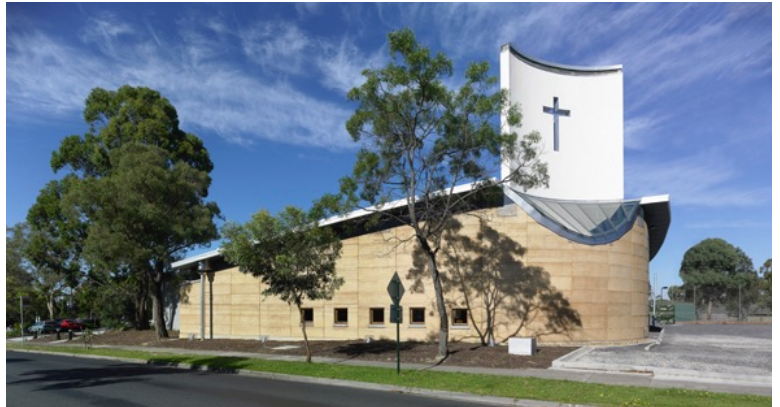
St Alfred's with thermal chimney and rammed earth wall
