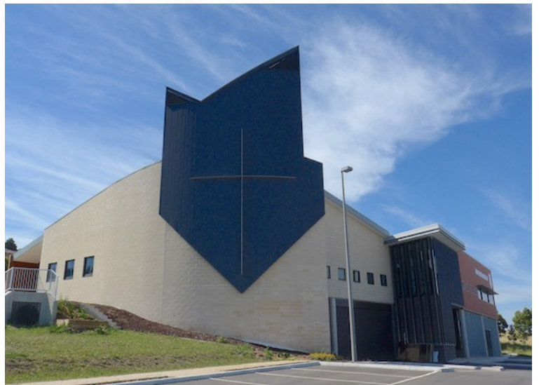
Obtaining all of the permits can take many months - the final facility can be a great help to mission, so start early . Mooroolbark Salvation Army Centre
